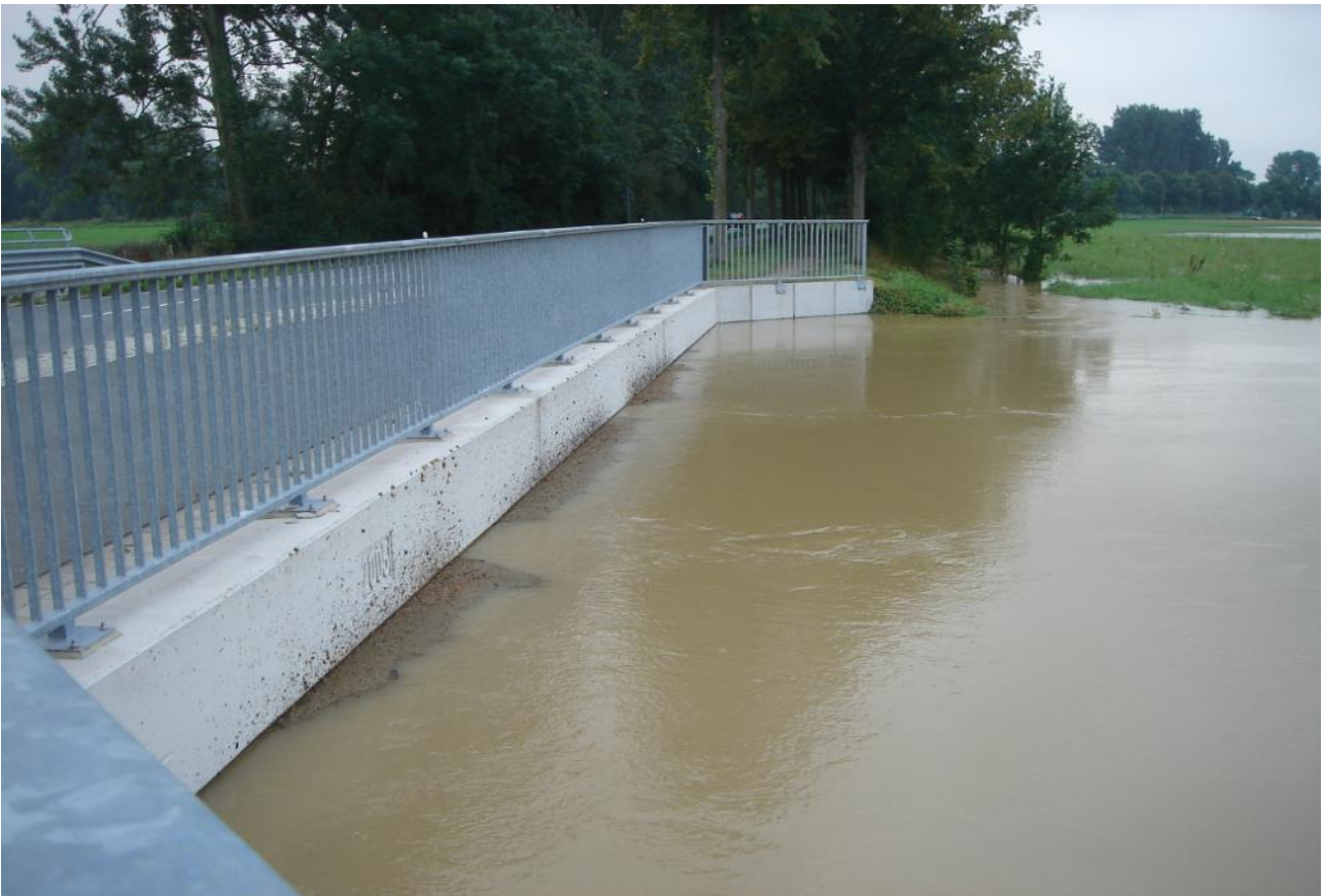
Flutbrücke Gieseler an der K42 in Lippstadt-Overhagen
